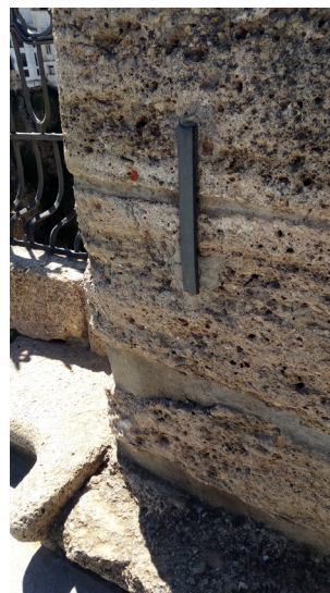
Figure 15. Clamp joining ashlar blocks in the parapet of the New Bridge (source: authors)
