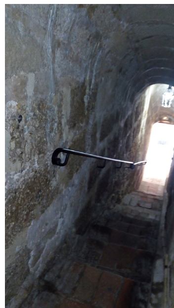
Figure 6. Gallery crossing one of the piers of the New Bridge (source: authors)
