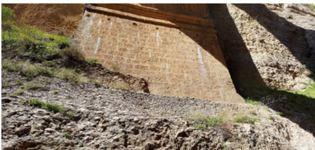
Figure 13. Foundation under the left abutment of the New Bridge (source: Lin, 2017)
