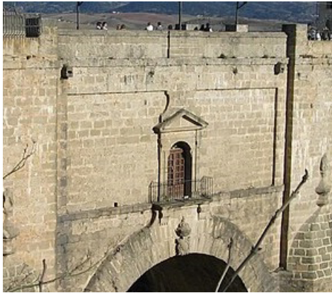
Figure 9. Balcony on central spandrel (source: Konstantin~commonswiki, 2025)
