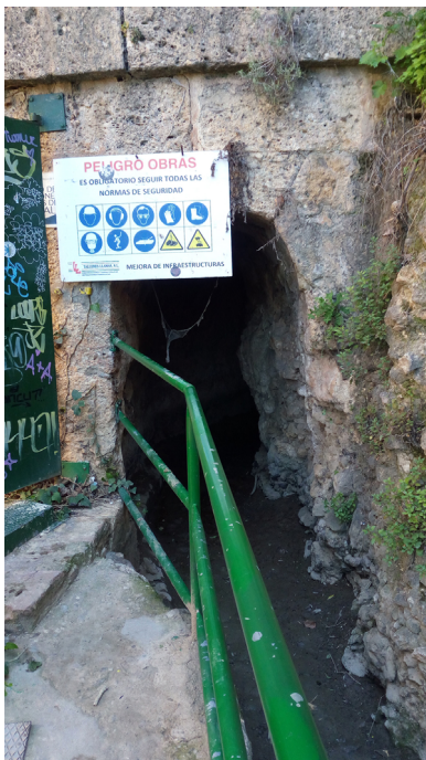
Figure 8. Access to the gallery located under the right abutment of the New Bridge (source: authors)
