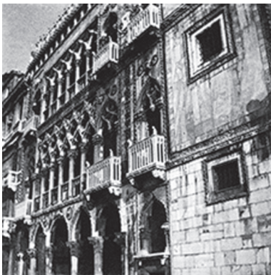
Fig. 4. Ch-E. Jeanneret, Façade of the Ca-d'Or's over the Canal Grande (1907). © FLC L4-19-15
