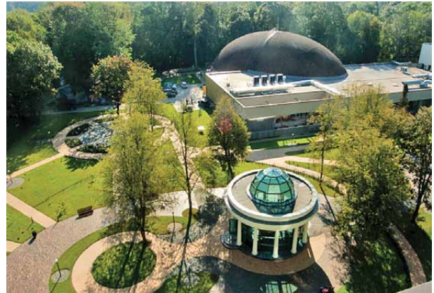
Fig. 11. Druskininkai "Grand SPA Lietuva" health and relaxation centre: the example of the innovative modernization of the urban complex in Lithuania
