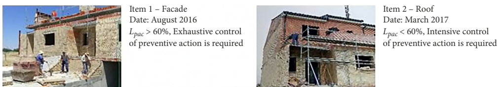
Figure 4. Images of the construction development of the work
